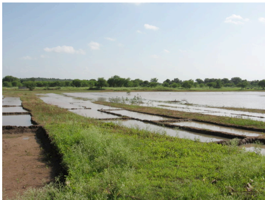
A typical NREGA worksite near Nalagonda village in Karimnagar, Andhra Pradesh. The ditches (known as “minor irrigation tanks”) help replenish the local water table by storing water from the monsoon that would otherwise runoff into rivers.
